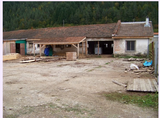
The building which will become our shelter/clinic.
